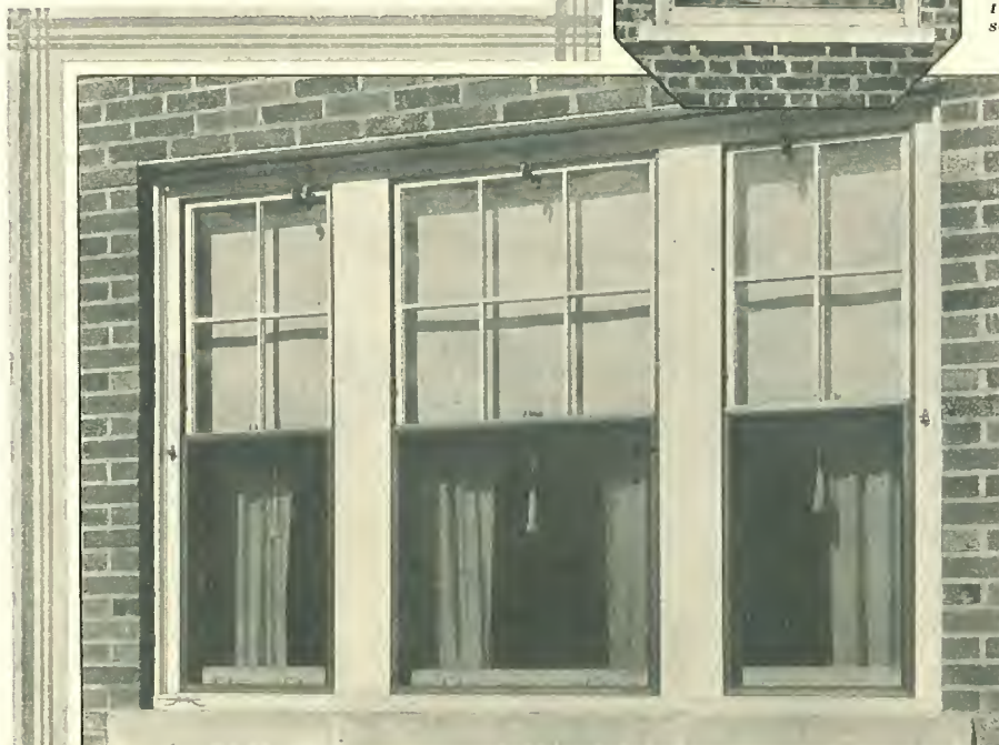
The channel guides in which vertical sliding screens operate are a permanent part of the window. They may be finished to match the trim color. Each window is numbered and corresponding number tacks are placed in sill. There is no difficulty in finding the right screen.
